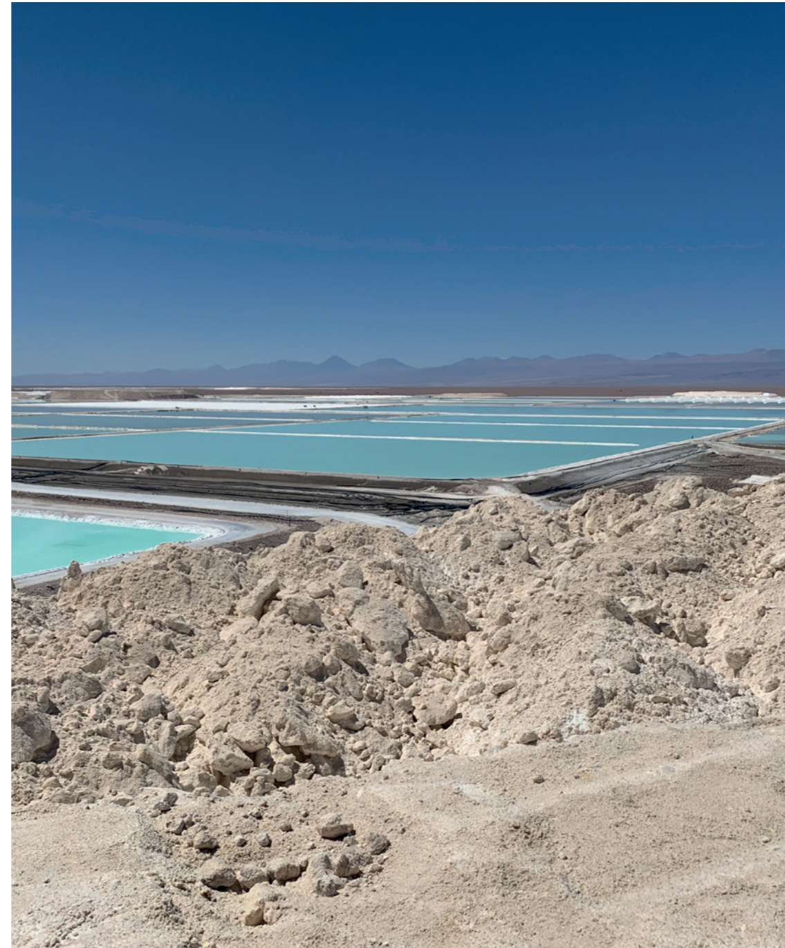
Evaporation ponds used for lithium extraction from salt flats in Chile.
